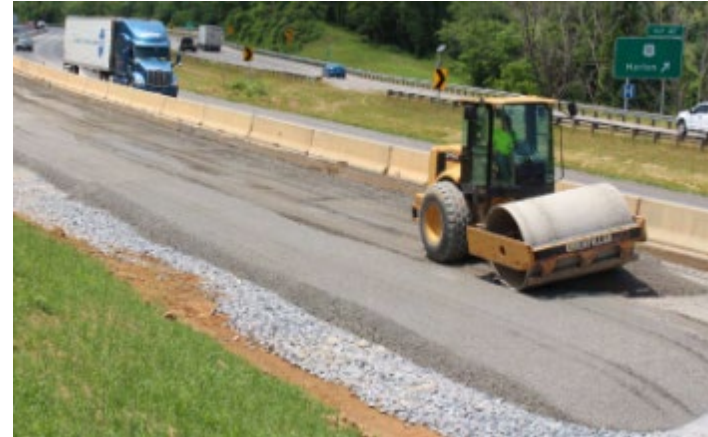
Exit 47 Smyth County
